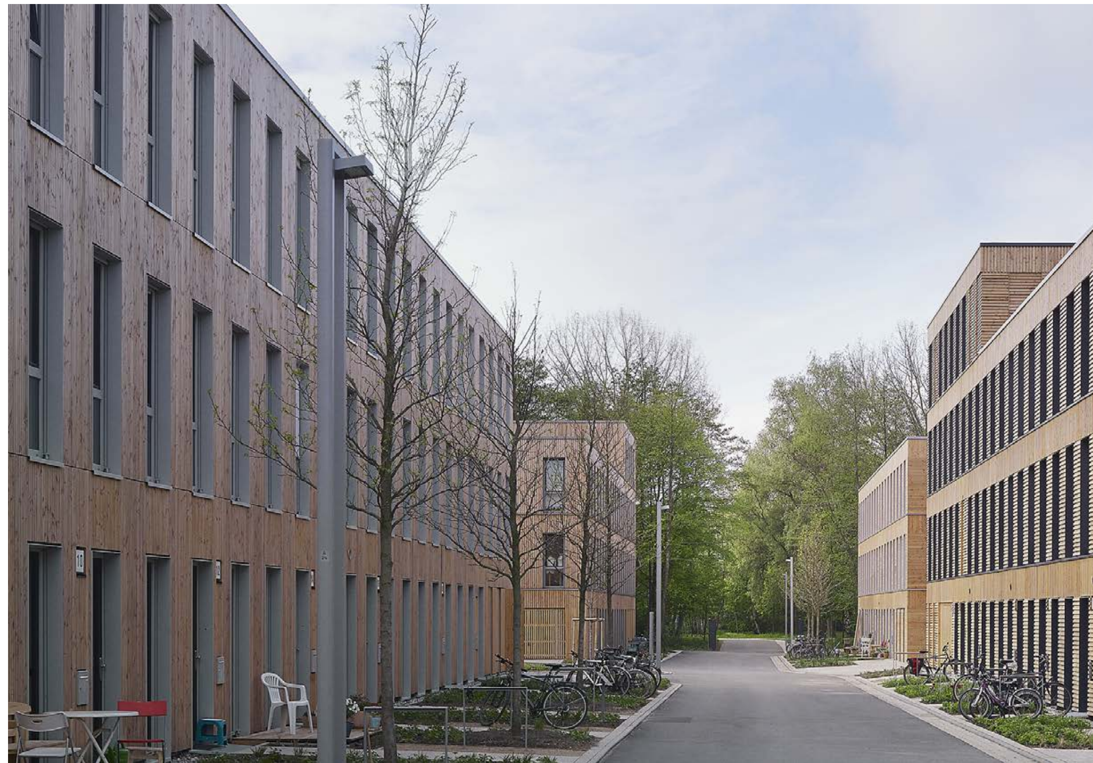
above: former view of the Falkenriedterrasse opposite page: view of Neue Hamburger Terrassen
