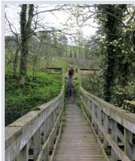
Footbridge at Newmill
