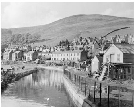
Walkerburn mill lade
