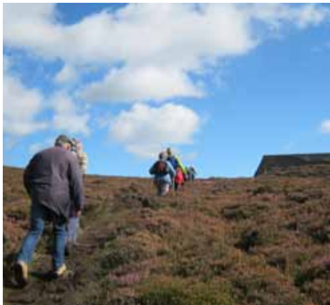
Approaching the water tank on Kirnie Law
