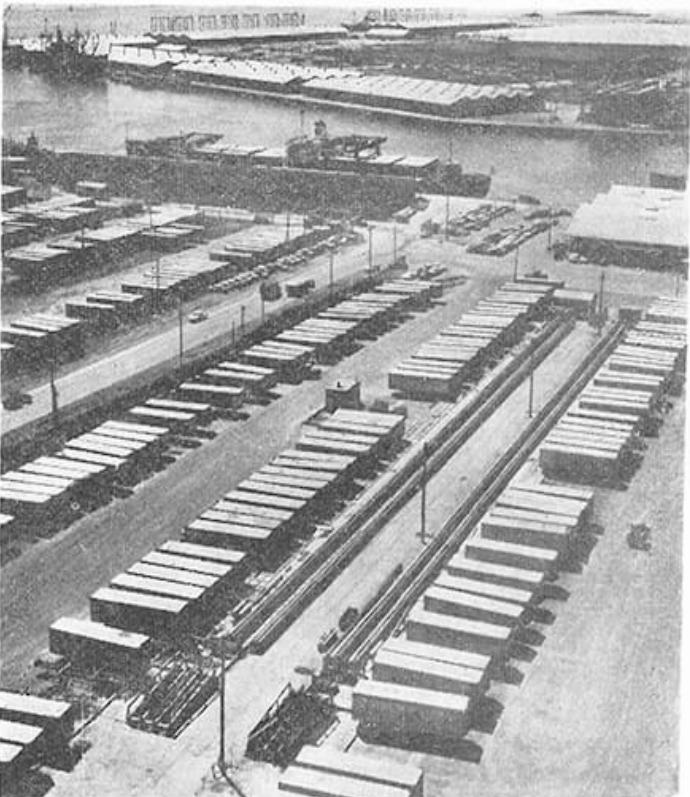
**CONTAINERIZED CARGOES:** The truck van containers shown here are a normal accumulation at the Sea-Land Service terminal at Port Newark, New Jersey. The vans are loaded by the ship's own gear.
