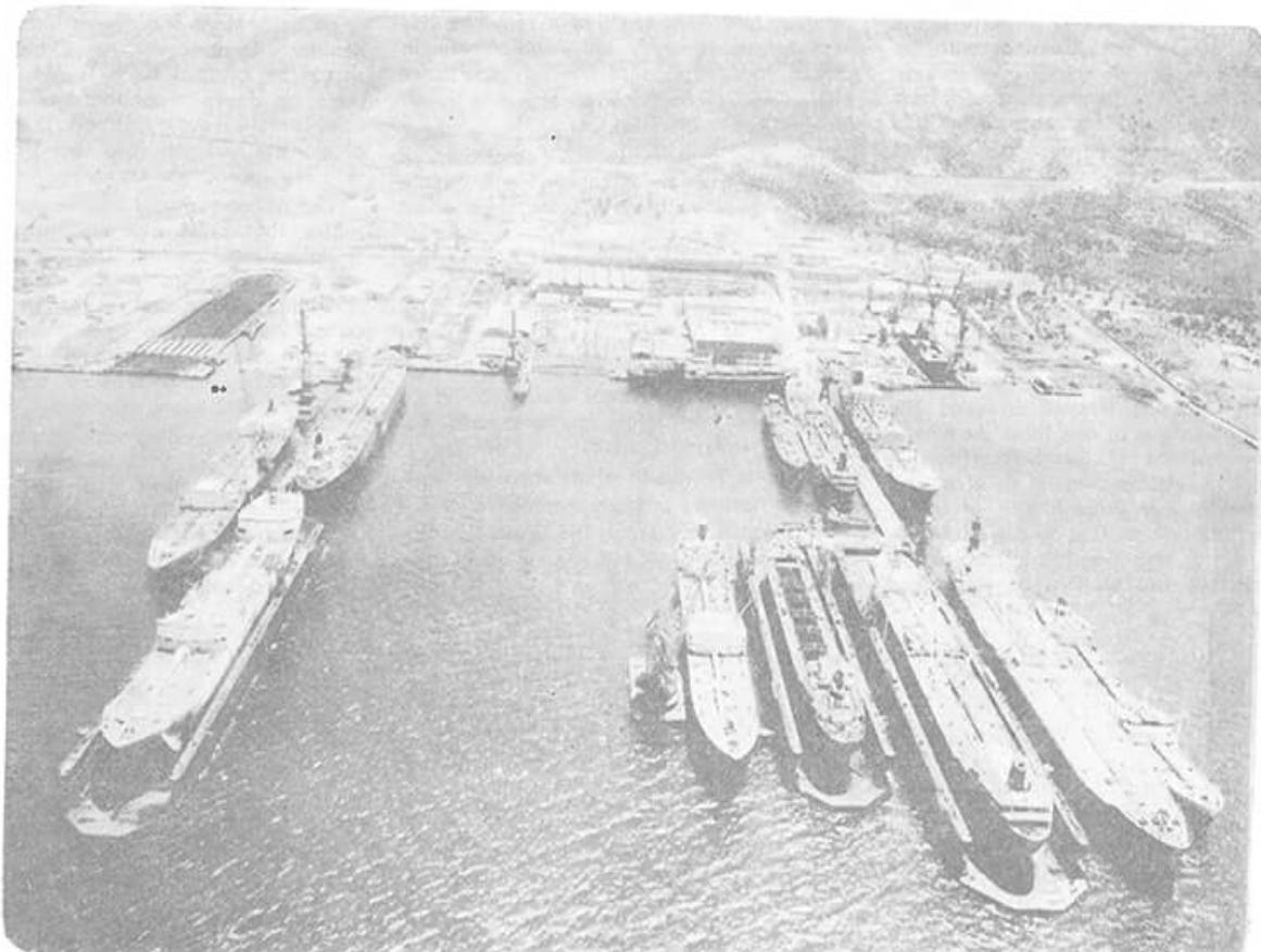
A general view of Skaramanga Yard with an S.D. 14 on building berth no. 1 at right. The 240.000-ton graving dock (under construction) can be seen at left.
