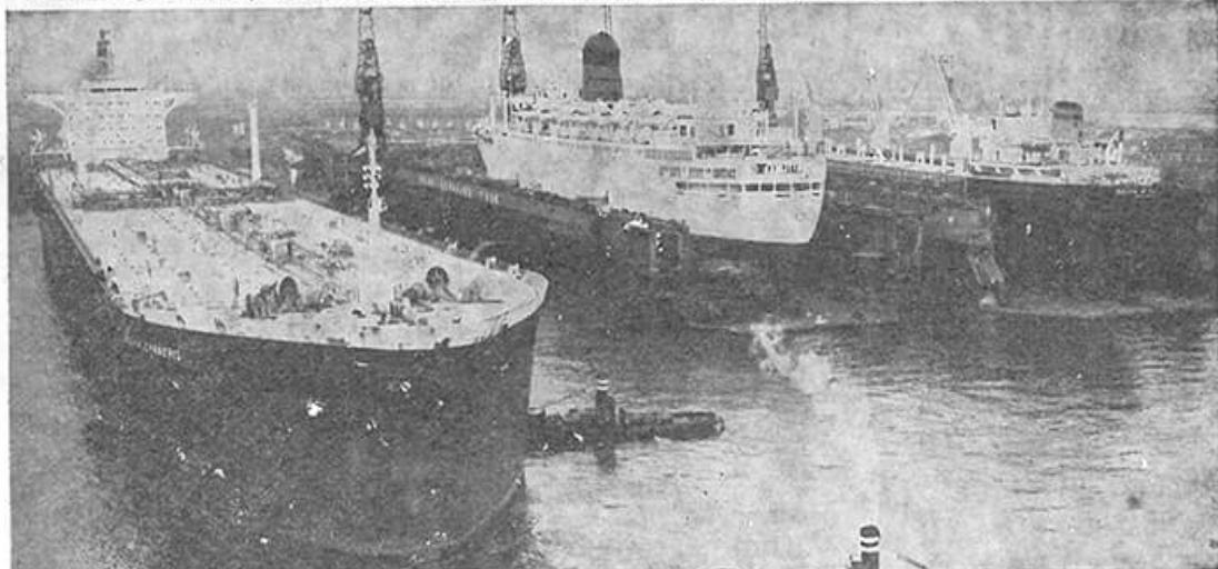
Nos. 9 and 10 floating dry docks of RDM capable of accommodating ships up to 100.000 dwt.
