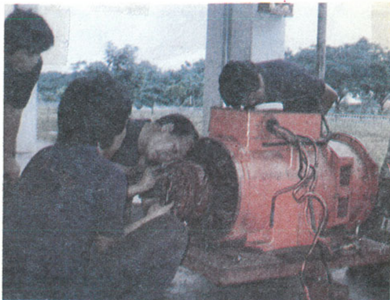
MOTOR REWINDING & ELECTRICAL WORKS
