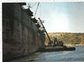
FLOATING WORKSHOP, SANDBLASTING
