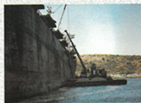
FLOATING WORKSHOP, SANDBLASTING
