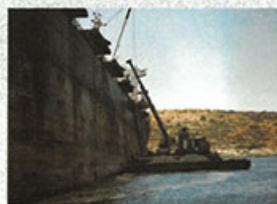
FLOATING WORKSHOP, SANDBLASTING
