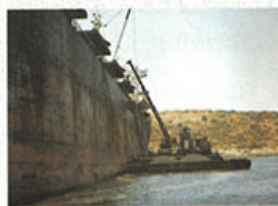
FLOATING WORKSHOP, SANDBLASTING
