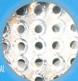
MAIN BOILER RE-TUBING
