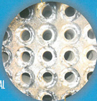
MAIN BOILER RE-TUBING
