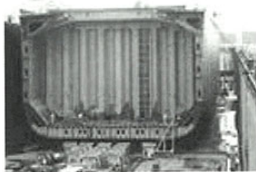
φωτο. 1. Construction phase of a double skin bulk carrier at Oshima
