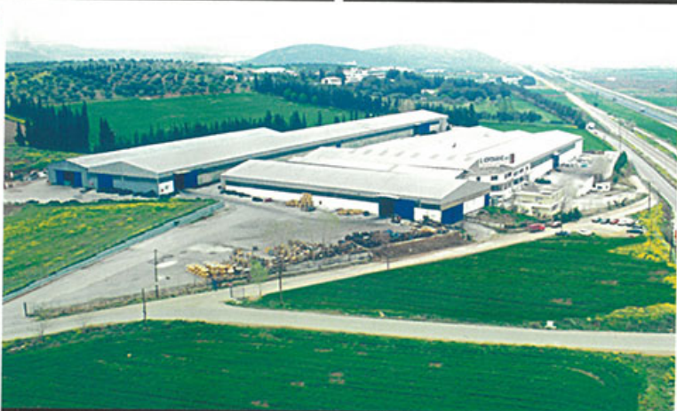
Manufacturing plant: more than 20.000m 2 of covered area
