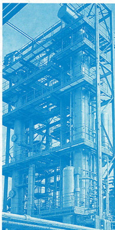
Two-column continuous rectifying plant built by Sulzer in Switzerland.
