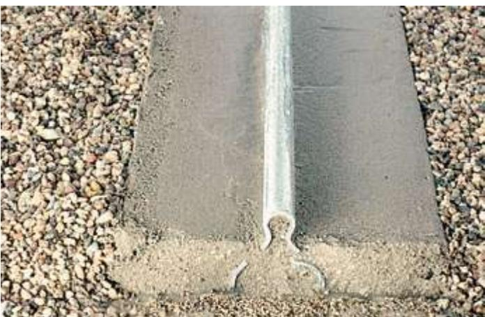
Make sure the gate was installed properly and check that the cement forms a single body with the track. Before installing the sliding gate, make sure that the cement has become solid.
