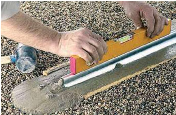
Once the track has been plunged into the cement casting, check with a level the levelness of the track, in order to assure a perfect movement of the gate.
