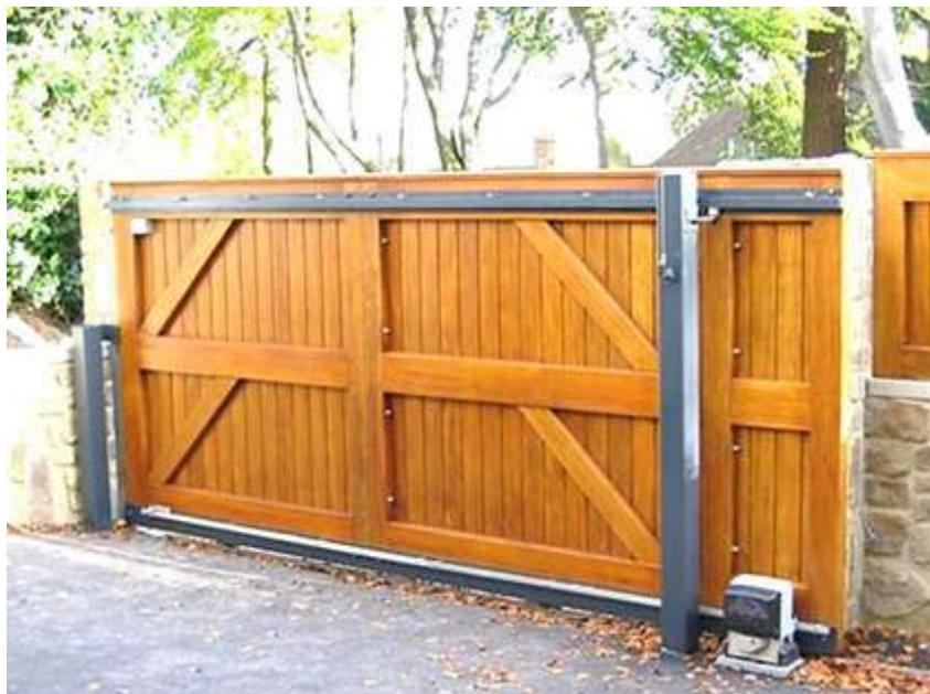
Supporting a gate in this way is good if you are converting a swing gate into a sliding. It may not be sufficient to install traditional hardware such as upper guide brackets or nylon rollers as there may not be the suitable posts in place.
