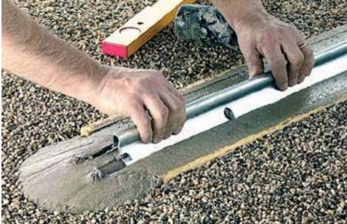
Plunge the track into the cement casting carefully verifying that it creates a single body with the same. The cement must necessarily enter in the whole internal part of the Profile; this will avoid noise production during the opening and closing of the gate.
