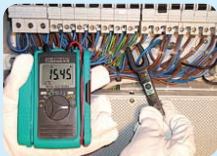
Measuring current in a Switchboard
