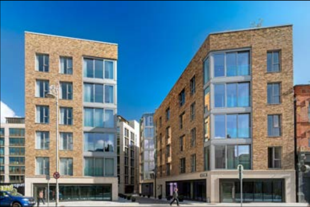
Richmond Street South Entrance Retail Units
