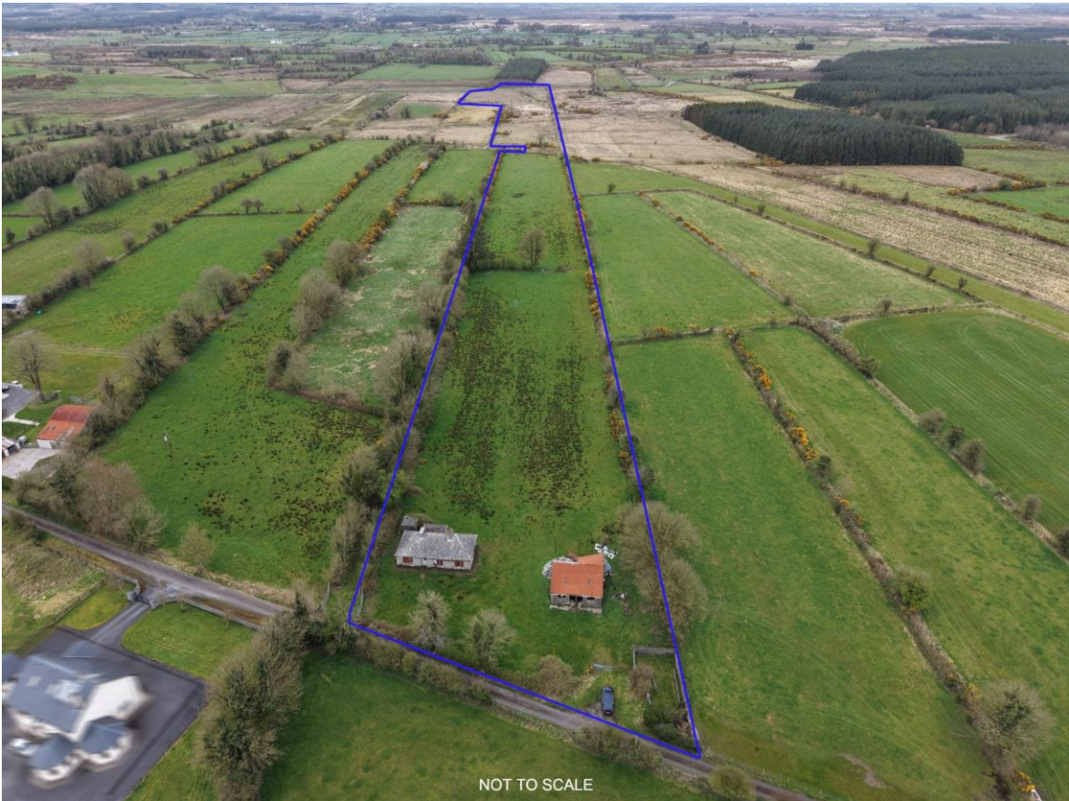
Derelict Residence On C. 14.40 Acres, Derryvode, Williamstown, County Galway
