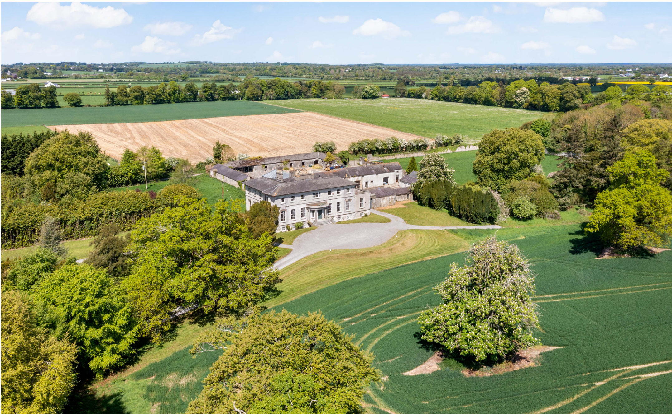
RATH HOUSE • APPROX. 882 SQ. M (9,494 SQ. FT) • 3 PRINCIPAL RECEPTION ROOMS • 7 BEDROOMS • 3 BATHROOMS • APPROX. 52 ACRES
