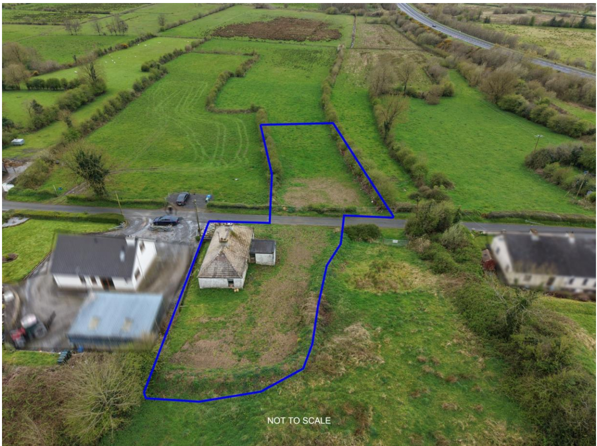
Derelict Residence, Ashbrook, Strokestown, Co. Roscommon
