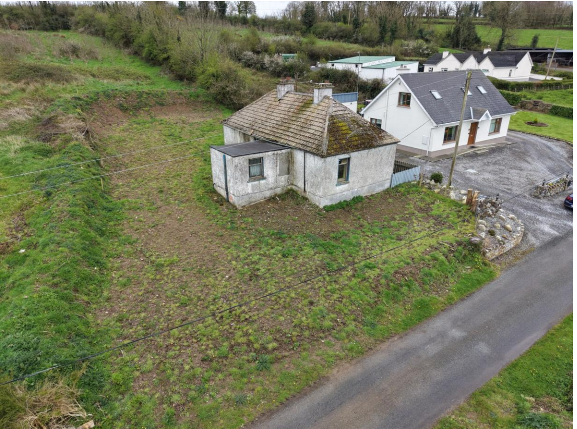
Derelict Residence, Ashbrook, Strokestown, Co. Roscommon
