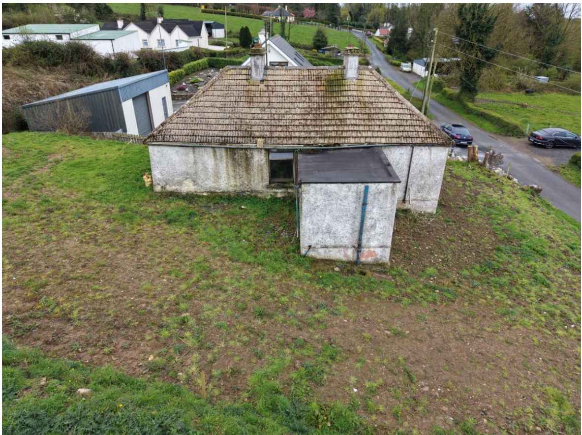
Derelict Residence, Ashbrook, Strokestown, Co. Roscommon
