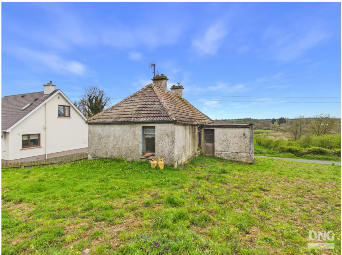
Derelict Residence, Ashbrook, Strokestown, Co. Roscommon
