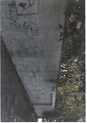
02 Boundary Wall A as Existing
