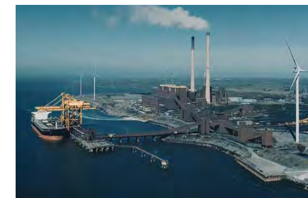
MONEYPPOINT POWER STATION
