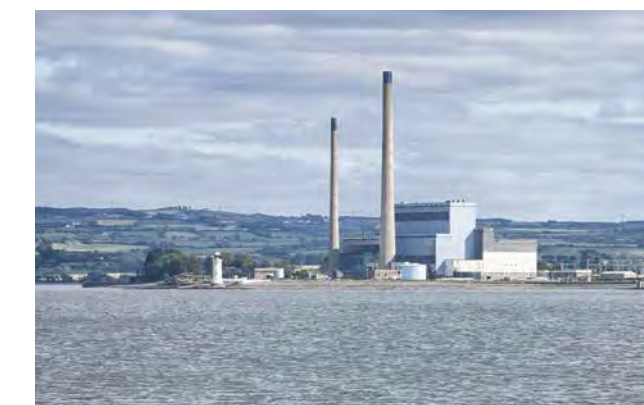
TARBERT POWER STATION
