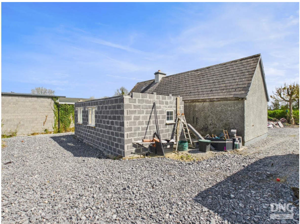
Rushestown, Newbridge, County Galway
