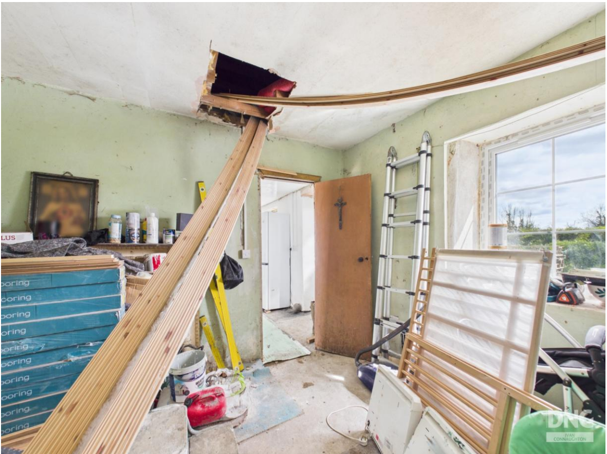
Rushstown, Newbridge, County Galway
