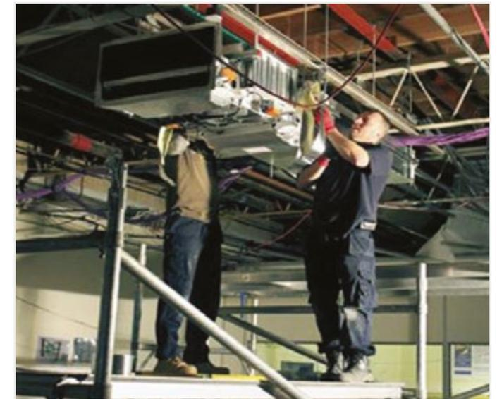
**Bryant Building Computer Room:** In January 2013 a computer room used by the Faculty of Science and Technology at Anglia Ruskin University in Cambridge had its aging air conditioning system replaced with two COOL-PHASE low energy cooling and ventilation systems. The units were fitted discreetly within the existing ceiling void.
