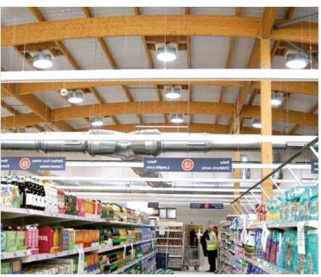
Sixty-four 750 mm diameter SUNPIPES® provide natural daylight for the shop floor with a further sixteen 750 mm diameter units fitted in the offices, and five 300 mm diameter units in other areas of the store.
