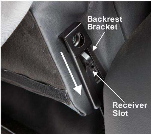
3. Position the backrest so its brackets sit on the receiver slot on both sides of the chair.
