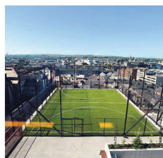
St Angela's is one of only a handful of schools in the country with a rooftop play space.
