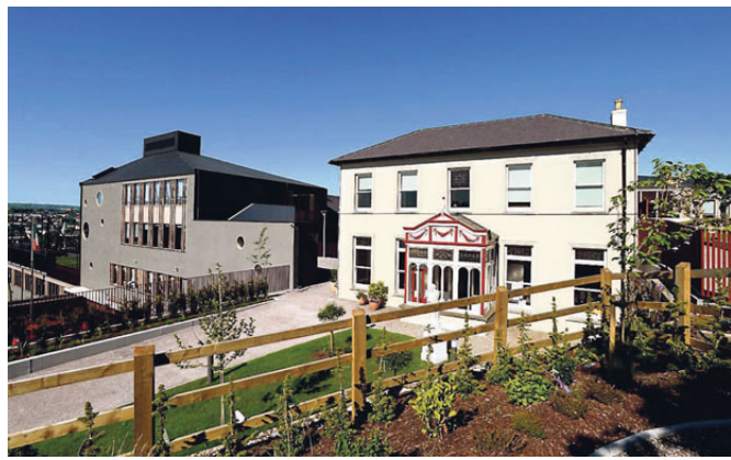
The old convent building stands in harmony with the new school building at St Angela's College in Cork.
