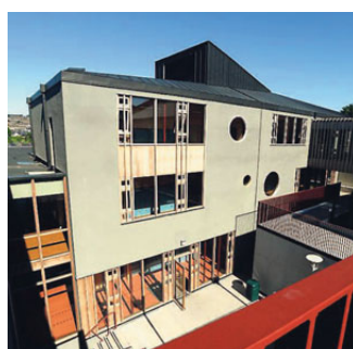
Internal circulation areas generally overlook active courtyards and teaching rooms look into quieter areas, or have views over the city.
