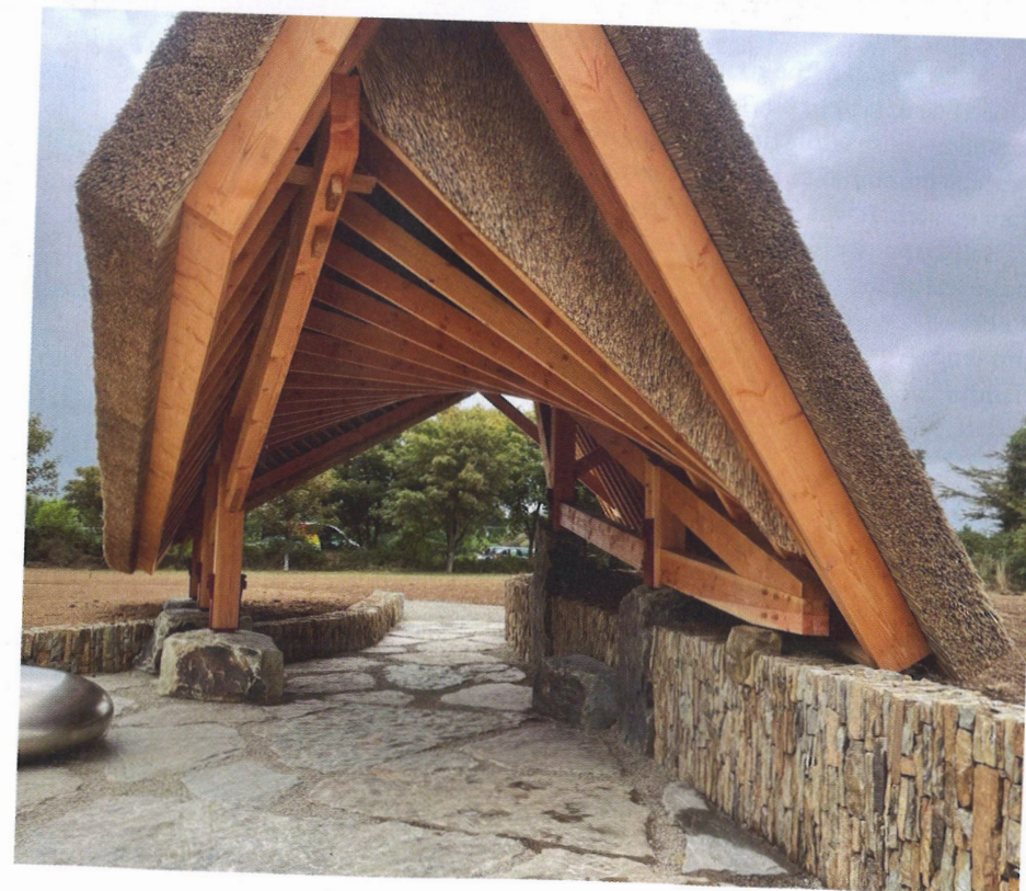
Below Passage House incorporates a flagged floor and stone piers from a nearby quarry, and dry stone walls quarried from the site.
