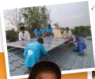
The BBOXX system links solar panels to a battery pack into which people can plug lights, phone chargers and televisions or power a space up to the size of a small office, depending on the size of the device.
