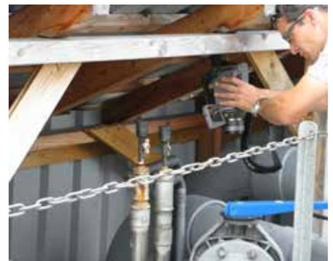
Engineer Ibeling van Lessen looking for gas leaks, which is possible from a safe distance and unusual angles using the FLIR GF320.
