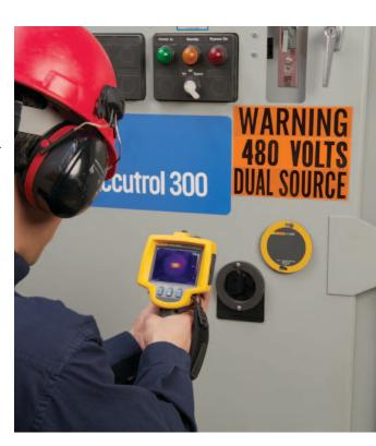
UL Recognized component. This allows the manufacturer to install IR Windows into their switchgear during assembly, prior to delivery to the customer without violating their UL Listing. As long as the IR Window is installed according to the IR Window manufacturer's instructions (instructions that are approved by UL during the UL5OV testing), the UL Listing of the switchgear is maintained.
