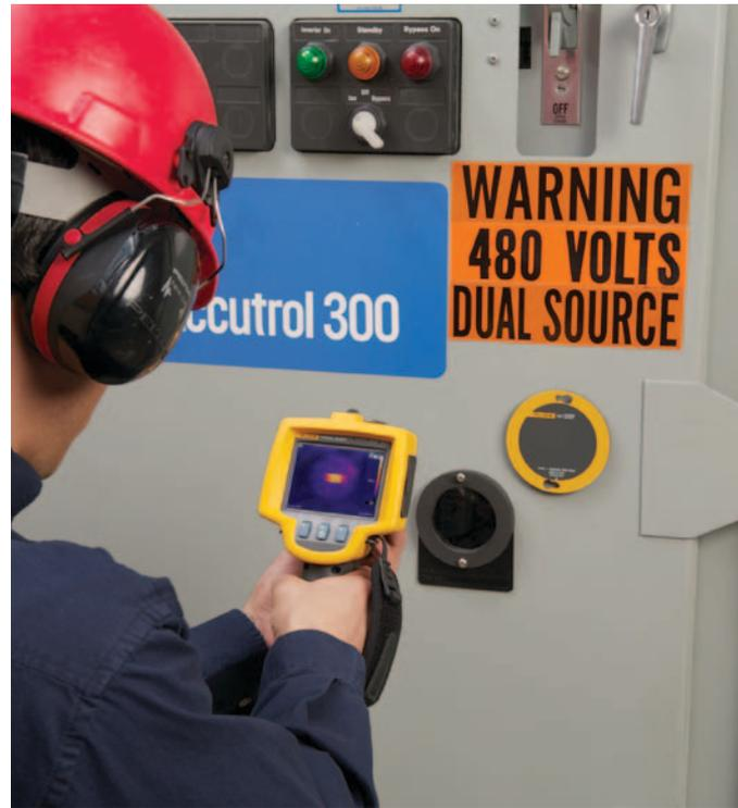
UL Recognized component. This allows the manufacturer to install IR Windows into their switchgear during assembly, prior to delivery to the customer without violating their UL Listing. As long as the IR Window is installed according to the IR Window manufacturer's instructions (instructions that are approved by UL during the UL50V testing), the UL Listing of the switchgear is maintained.
