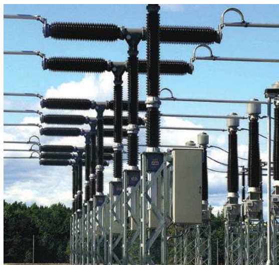
Disconnecting circuit-breaker. Same contacts for switching and disconnecting functions.
