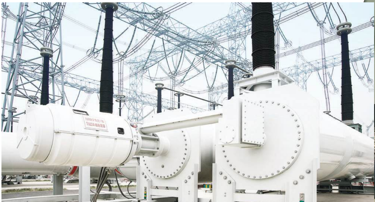
Circuit breaker, 1000 kV
