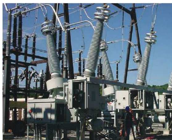
Dead tank circuit breaker
