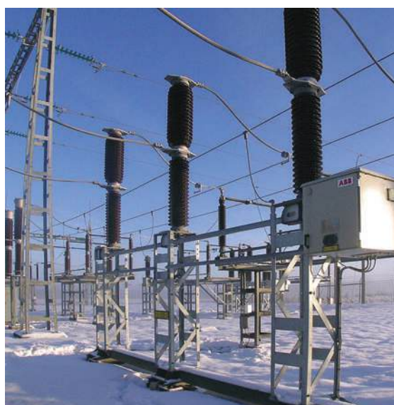
Live tank circuit breaker
