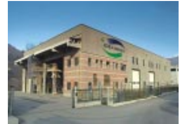
The new IDEA GRANDA plant, in the Province of Cuneo, Italy.
