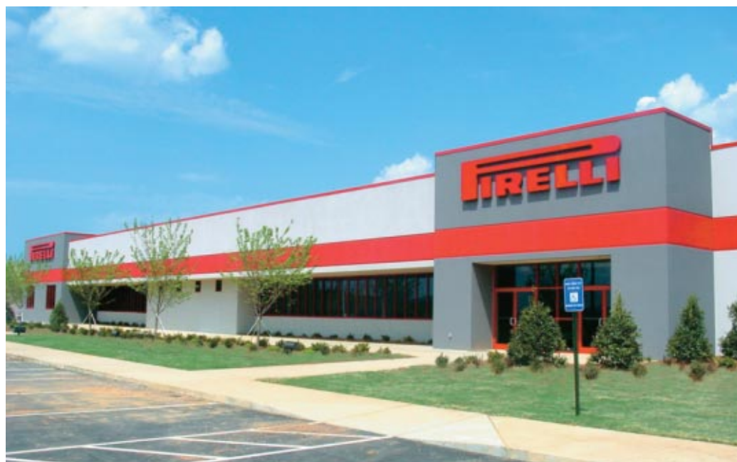
The first MIRS™ factory overseas went into operation in Rome, Georgia (United States).
