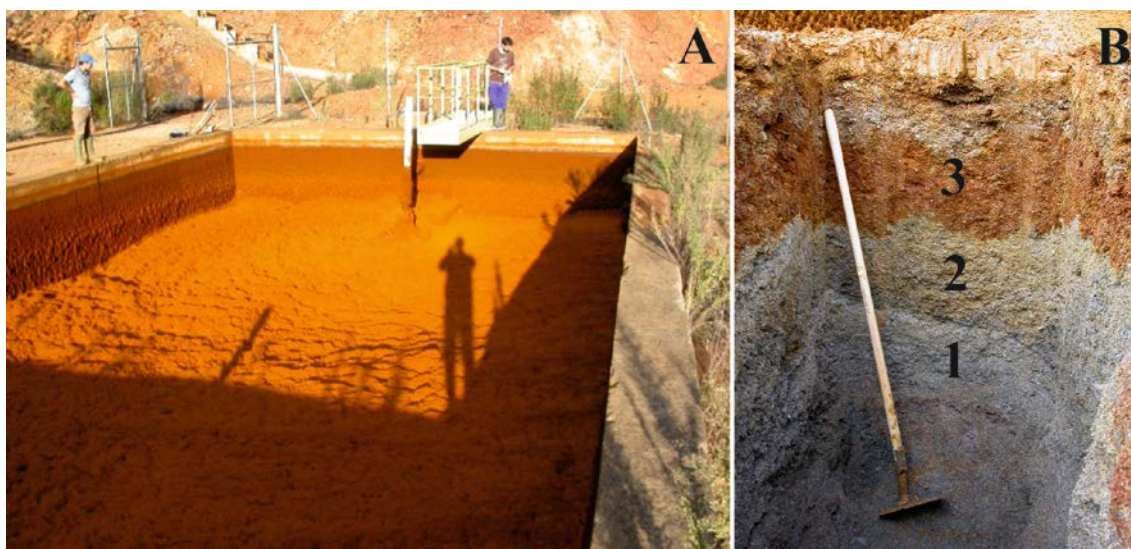
Figure S19-S6. A) View of the Mina Esperanza passive remediation systems after 15 months of functioning. B) Detail of the vertical zonation: calcite-gypsum (1), basaluminite (2) and schwertmannite (3) zones.
