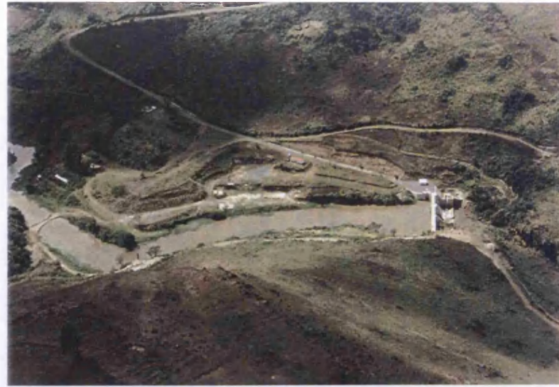
2. Dam on River Turasha, the main tributary of River Malewa.
