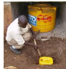
**Photograph 4. Urine collecting mechanism**
