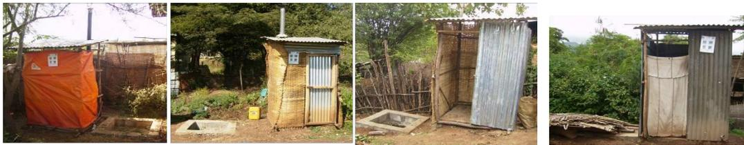
**Photograph 6. Fossa alternas constructed with different material**
