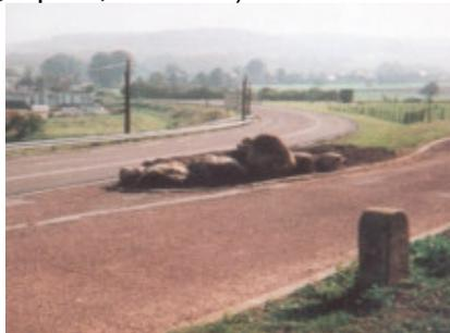
Figure 19: Example of boulders in the roadside safety zone
