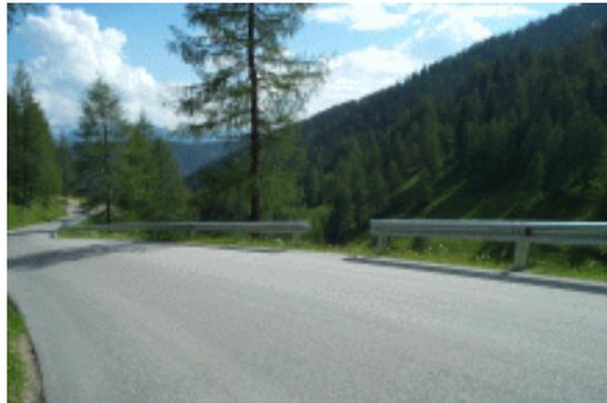
Figure 17: Gaps in guardrail
