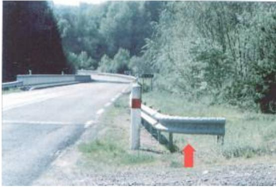
Figure 18: Guardrail termination
