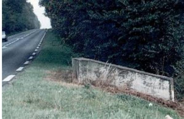
Figure 13: Culvert headwall
