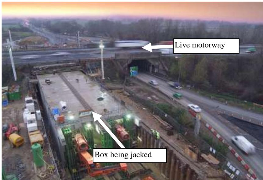
Figure 1. RC Box-Jacking under a live motorway
