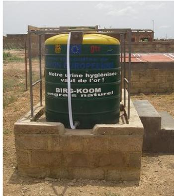
**Figure 5. Plastic urine storage tank in Ouagadougou, Burkina Faso installed as part of EU-funded project ECOSAN\_UE, Sept. 2008**
