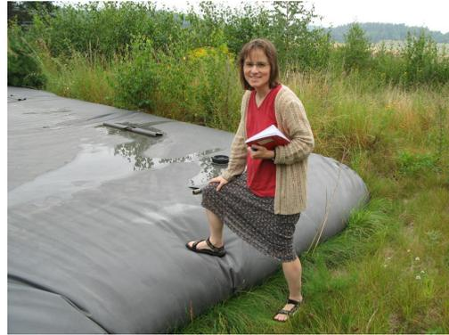
**Figure 6. Urine storage tank made of a PVC bladder (3 x 150 m<sup>3</sup>) at Lake Bornsjön near Stockholm (Sweden), Aug. 2007**
