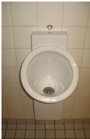
**Figure 1. Waterless urinal of Keramag, Germany (model Centaurus).**
