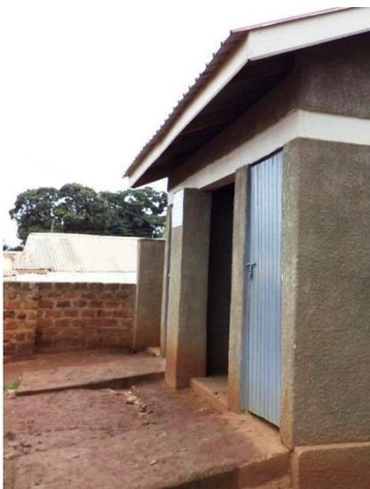
**Photo 1.** Ramps with gradient 1:12. Note lack of platform at top of ramp and high door bolt. This would be inaccessible for a wheelchair user. (Kasumba 2012)
