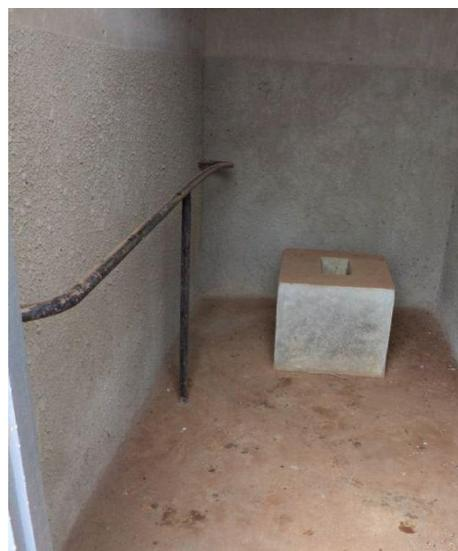
**Photo 2.** Cubicle with raised toilet seat and support rail. The space inside looks adequate, but the inward opening door (see photo 1) reduces the usable space. (Kasumba 2012)
