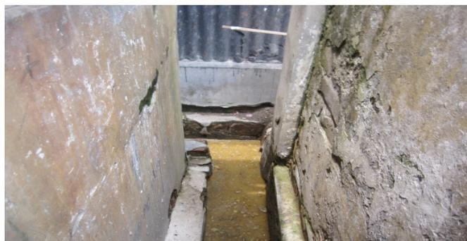
**Photograph 1. Direct discharge of sludge from containment**
