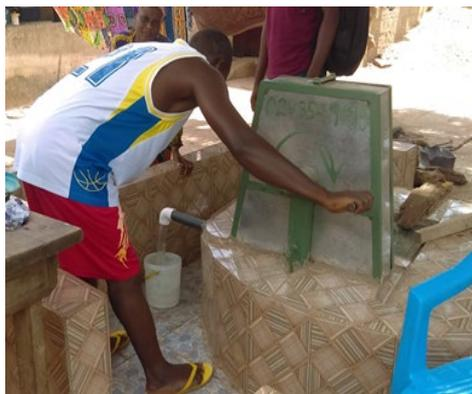
Owing to perennial piped water supply shortages, one household head, a retired agriculture extension officer, invested in the construction of a 16m-deep well, lined and fitted with a hand pump. Although the household has a piped water supply yard connection, the lined well is the primary water source. Water flow is continuous and reliable during normal weather but becomes less reliable during extremely hot conditions.
