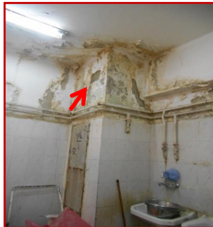
Photos of deteriorated paint samples collected from different sites in Assiut University hospitals.
