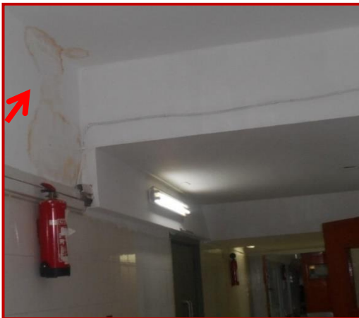
Photos of deteriorated paint samples collected from different sites in Assiut University hospitals.
