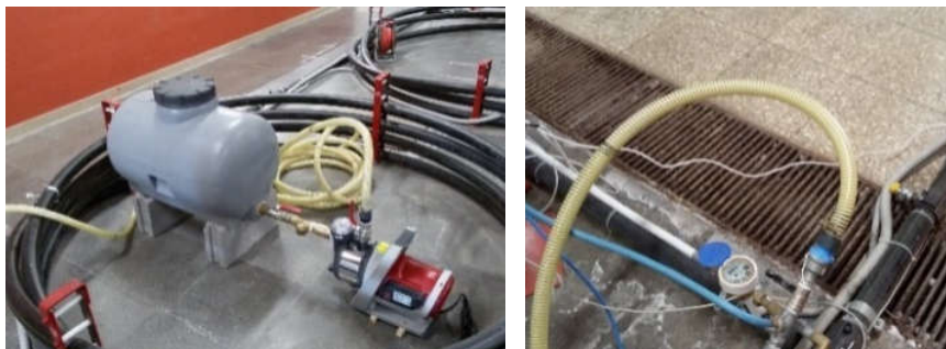
Figure 3. Installation of the pump-reservoir system (left) and connection to node (right).
