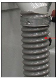
Check the extraction hoses for holes or breaks as these will affect the rate of extraction from the cabinet.
