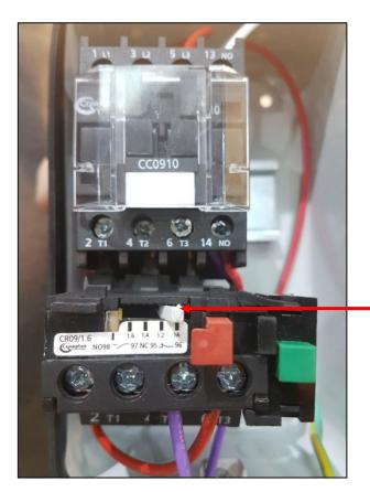
To adjust, pull out selector and slide to required position
