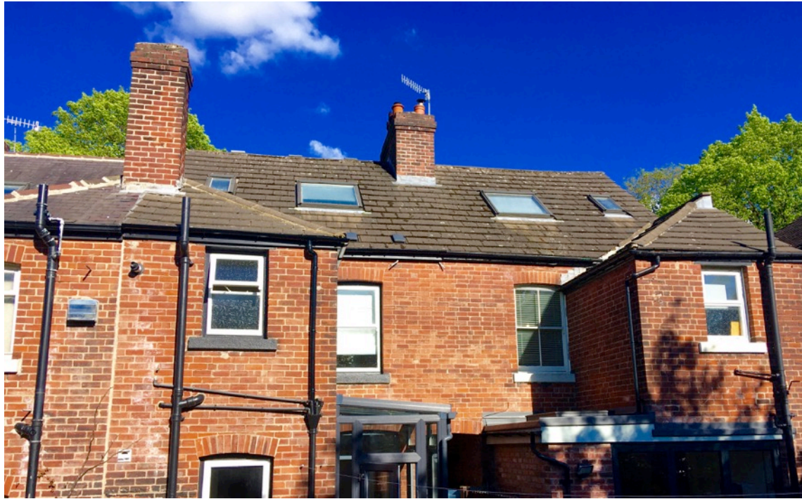
Note that unlike the terrace in the previous photograph the party wall in these Victorian houses is not taken above the roof-line.
