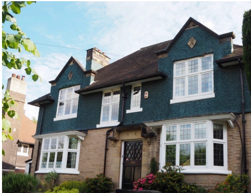
Edwardian houses tended to have casement windows especially those more obviously associated with the Arts and Crafts movement (bottom image).
