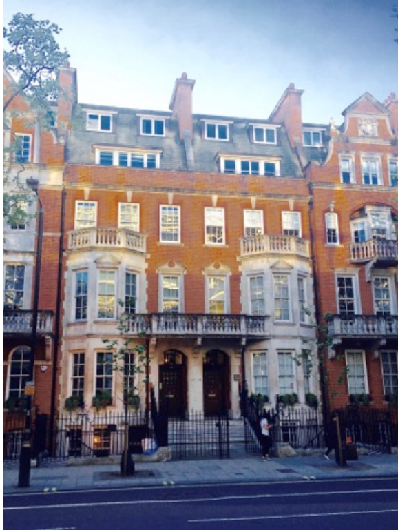
This photograph shows a mansard roof to an Edwardian dwelling.
