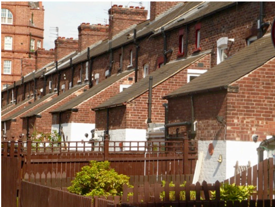
The courtyards to these working-class houses have been turned into gardens following a regeneration scheme in which neighbouring terraces were demolished.
