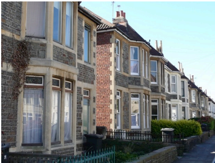
This photograph shows a common arrangement of a rubble façade with brick walls to the side elevation. Bricks would also have been used on the inner skin of the stonework and the rear walls. Sometimes the brick would be covered with render.
