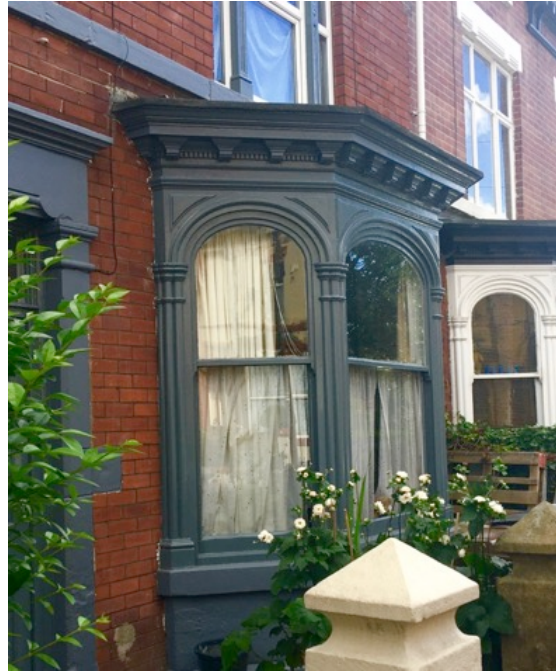
Single story bays might have a parapet and a flat lead roof as in the photographs above or a pitched roof as shown in the previous photograph.
