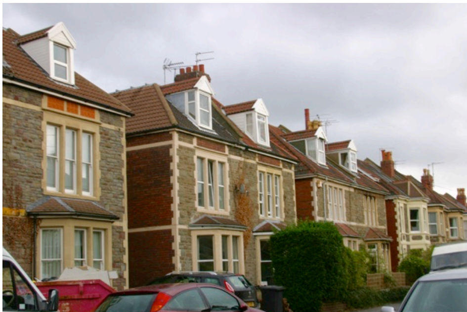
The hipped roofs of these semi-detached houses are covered in double roman tiles– some are still the original clay but others have been replaced with concrete versions.
