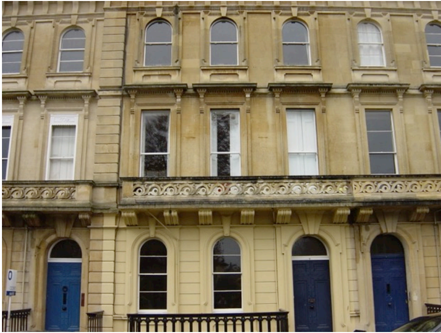
This terrace of houses, which could be mistaken at first glance as being Georgian, was constructed well into the Victorian period (1875).
