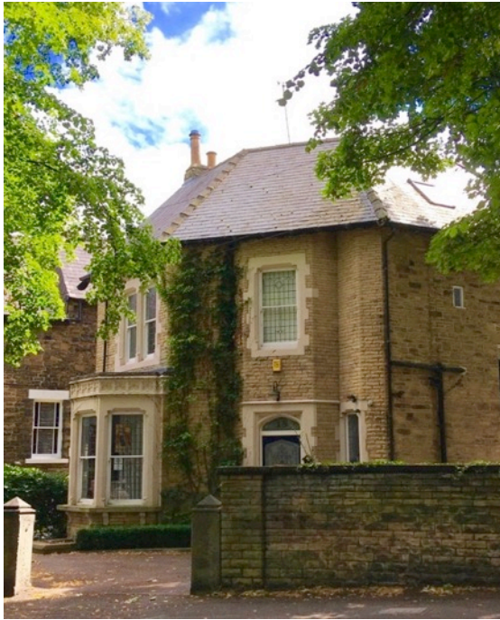
Single story bays might have a parapet and a flat lead roof as in the photographs above or a pitched roof as shown in the previous photograph.
