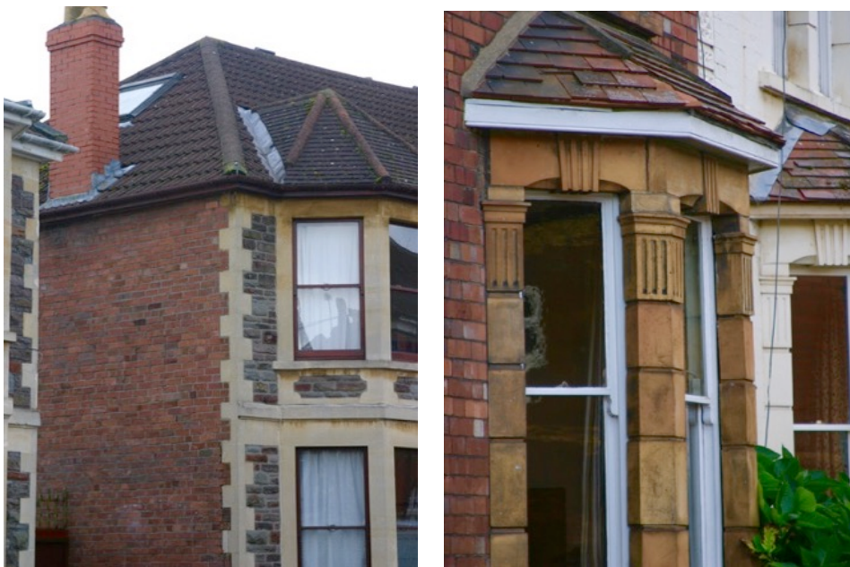
A double storey bay constructed in ashlar limestone and a single storey bay in terracotta (both with sliding sash windows).
