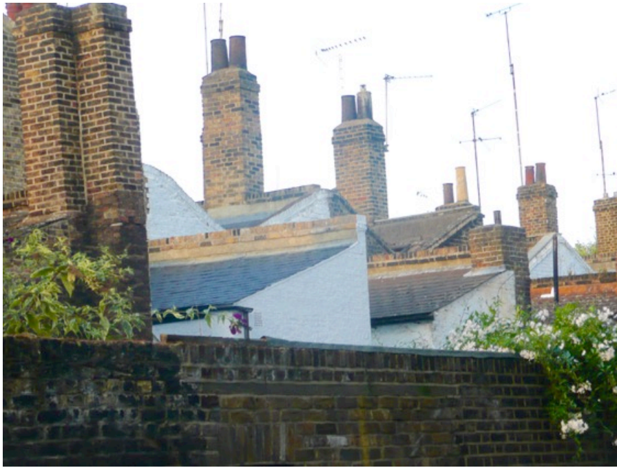
This photograph is a view to the rear of rather typical working-class houses with a rear annexe (usually referred to as a back addition or offshot).
