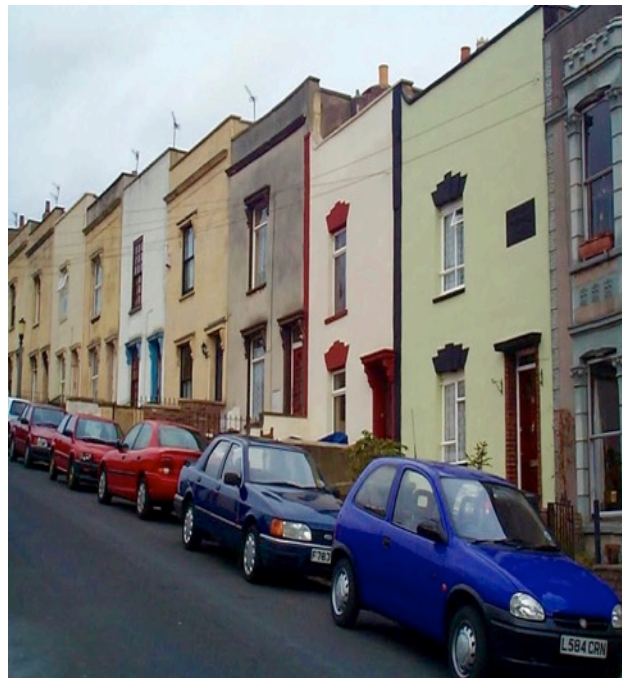
Note that unlike the terrace in the previous photograph the party wall in these Victorian houses is not taken above the roof-line.
