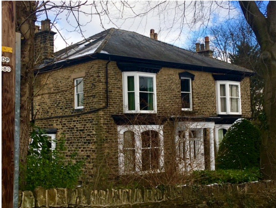
The hipped roof of this detached house has a slate roof covering.
