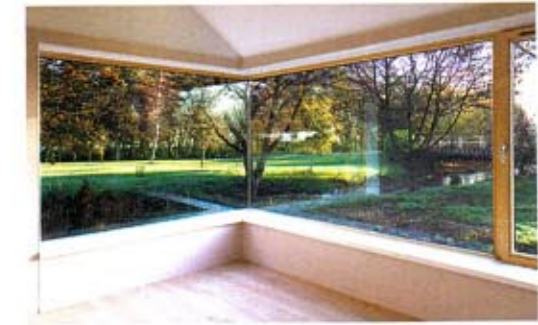
In the dining area, which floods with light in the afternoon, a cantilevered corner window measuring four by eight metres frames views onto the river.
