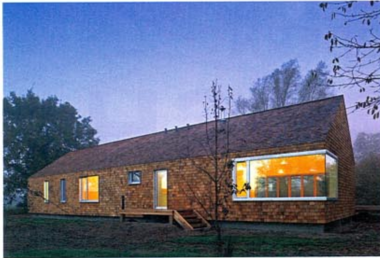
The house is clad in 15,000 untreated cedar shingles, a material that belies the prefabricated system beneath. Fixed to battens over a breathable waste wood chip building board, cedar was chosen as a cost-effective alternative to weatherboard.
